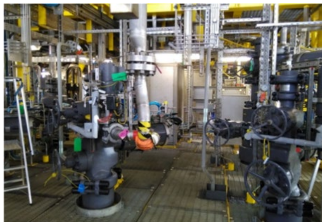
TWB Wells Hook-up complete
